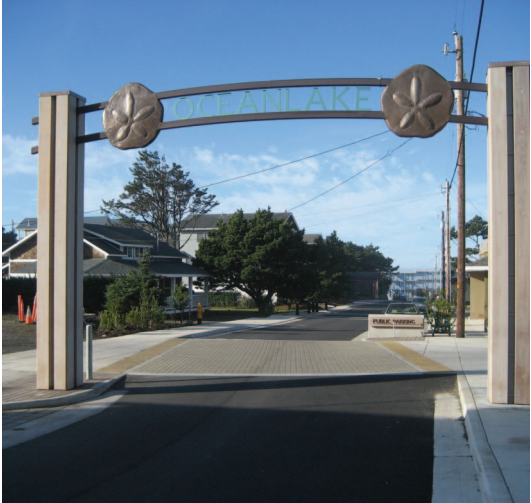
NW 15th Street Streetscape
