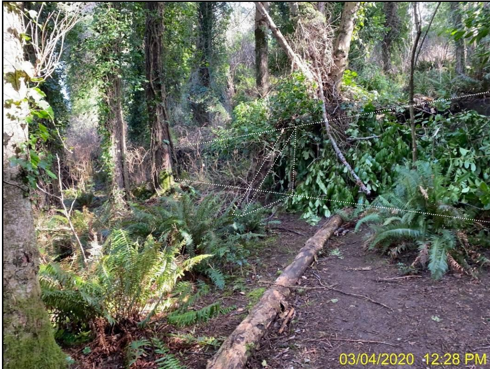
Photo 8: Lower driveway area with buttressed retaining wall covered in vegetation.
