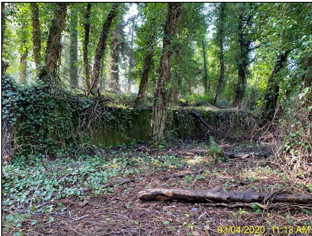
Photo 1: Upper area, terraced with retaining walls (near TP-5).
