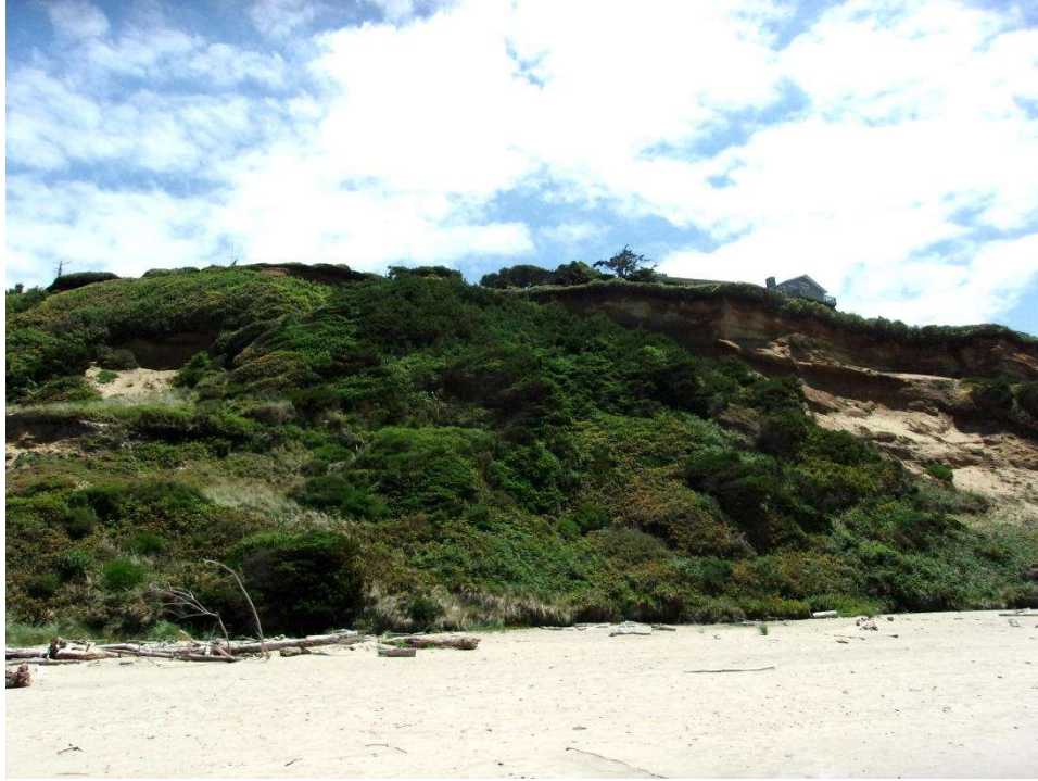
Photo 5 – Easterly view of the bluff slope, west of the subject site.
