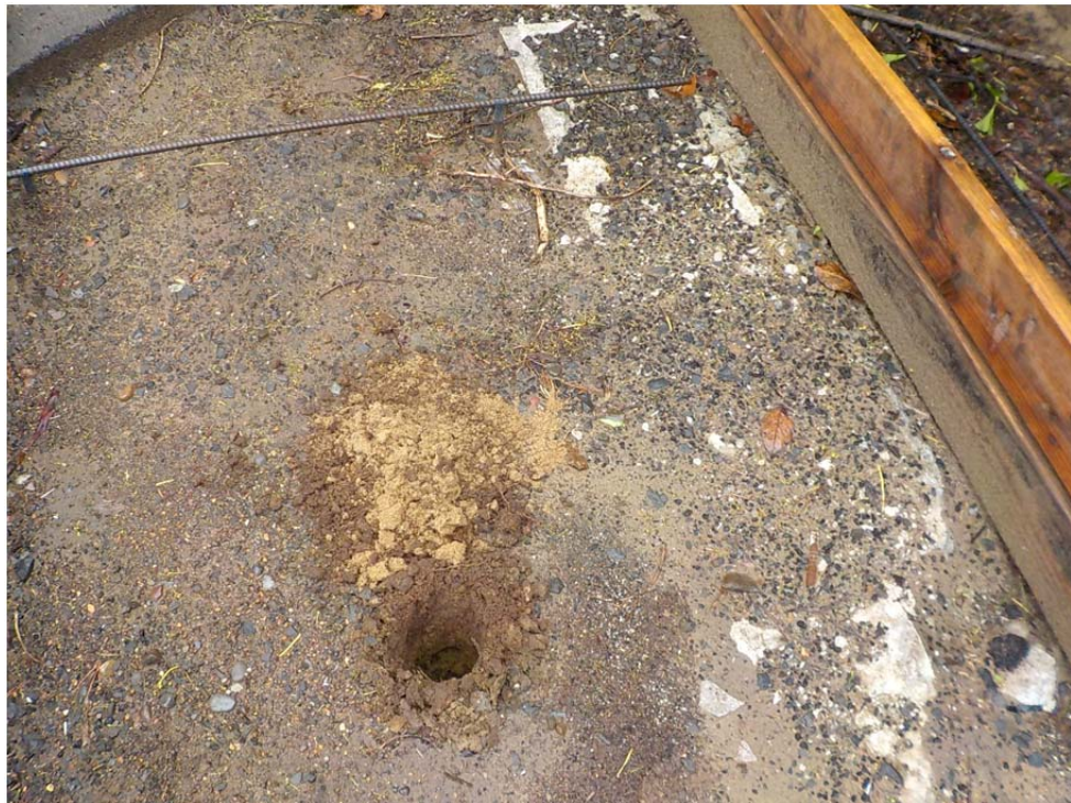
Photo 4 – View of the soils encountered in boring B-3.
