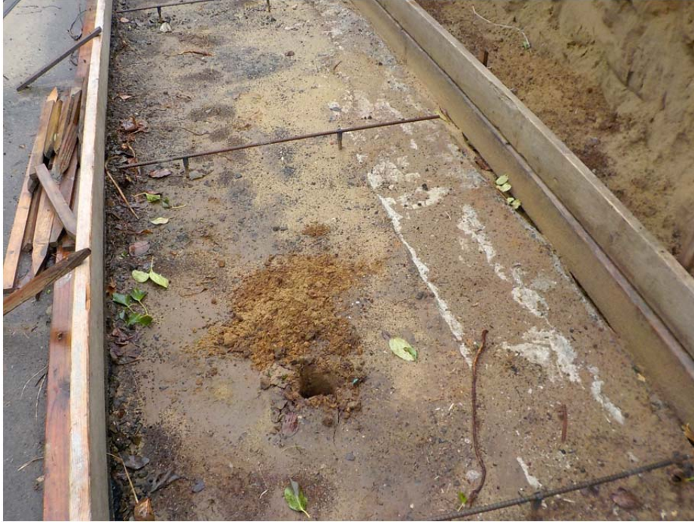
Photo 3 – View of soils encountered in boring B-1.
