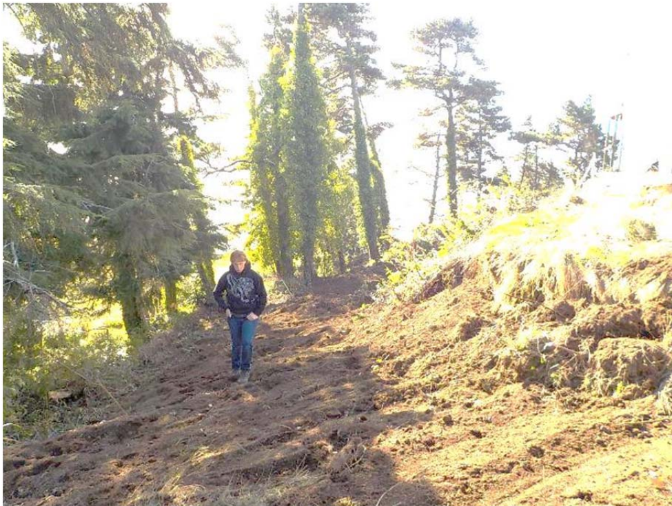
Photo 14 – View of the disturbed ground surface from grading activities on Tax Lot 1800 (10/31/2019).
