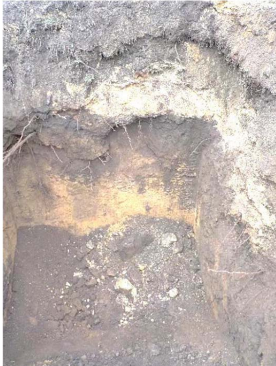
Photo 20 – View of the native dense sand underlying organic-rich soils and fill exposed in the test pit (04/05/2018).
