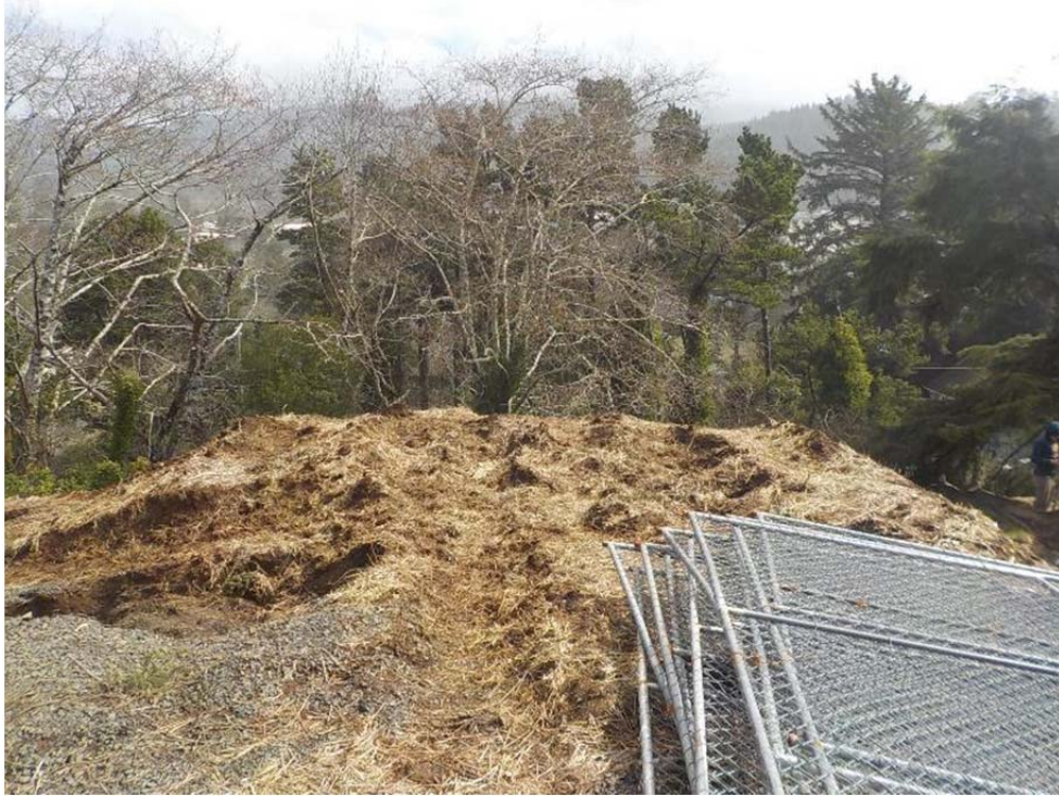
Photo 11 – Easterly view of the large fill stockpiled on Tax Lot 1300 (3/22/2022).
