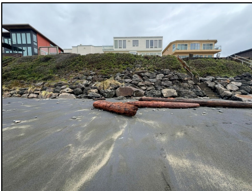
Photo 1: Adjacent beach, looking east toward the existing residence and revetment.
