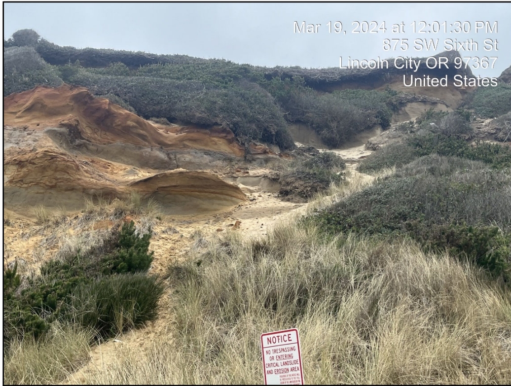
Photo 6: View of the sandstone bluff on western edge of property, with notable landslide warning sign at the base of the bluff.
