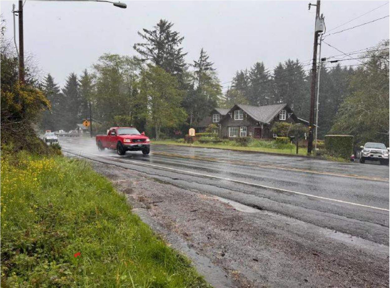
Figure 7b. View toward Southbound US 101 from the realigned access showing that regrading of the hillside will be required to obtain adequate sight lines. Regrading and widening will occur to support the new left-turn lane and sidewalks along US 101 as part of site frontage improvements.
