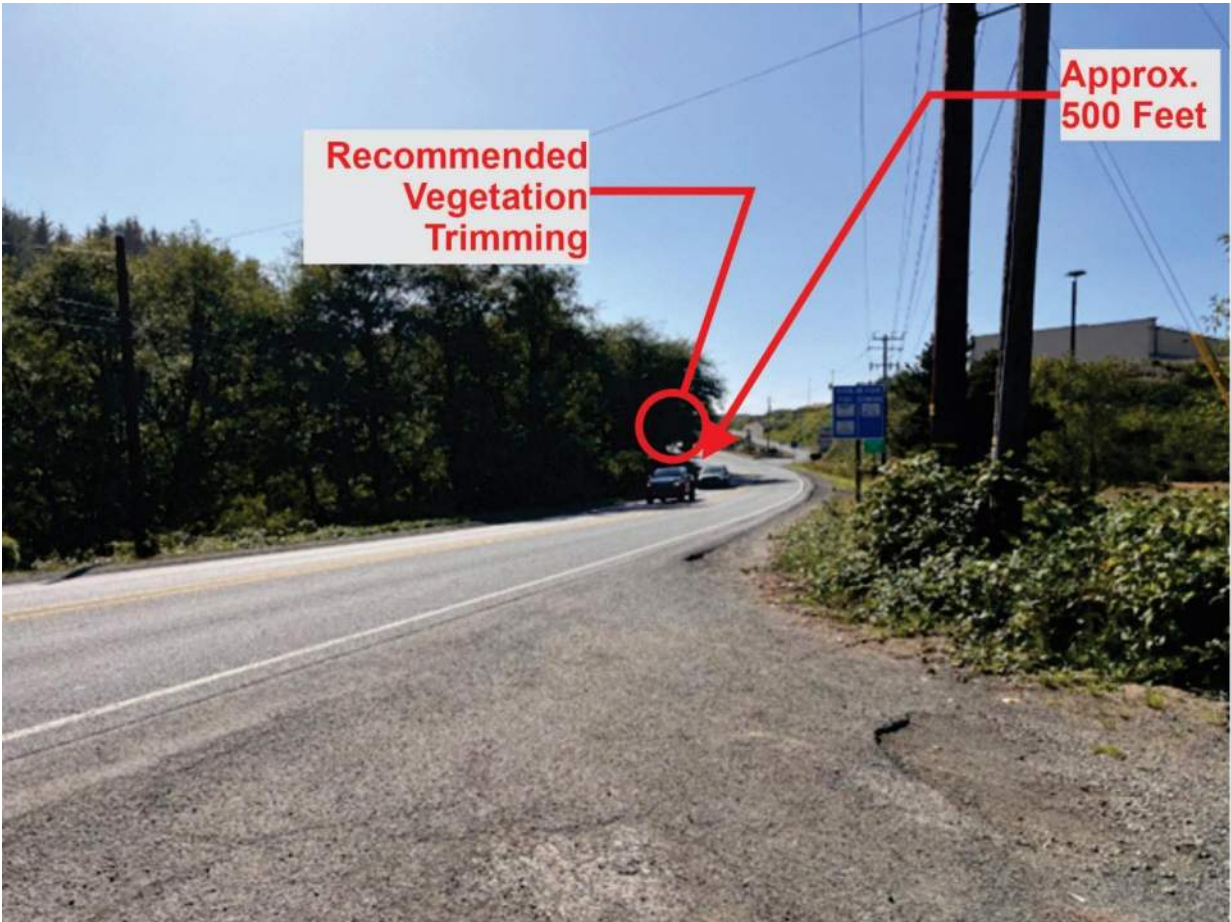
Figure 6a. Existing view from the residential driveway facing toward northbound US 101. The figure shows that the full width of the Lighthouse Square access is visible; trimming of vegetation within highway right-of-way along the curve and relocation of the tourist information sign would be necessary to provide the recommended 530-foot AASHTO-recommended sight distance.
