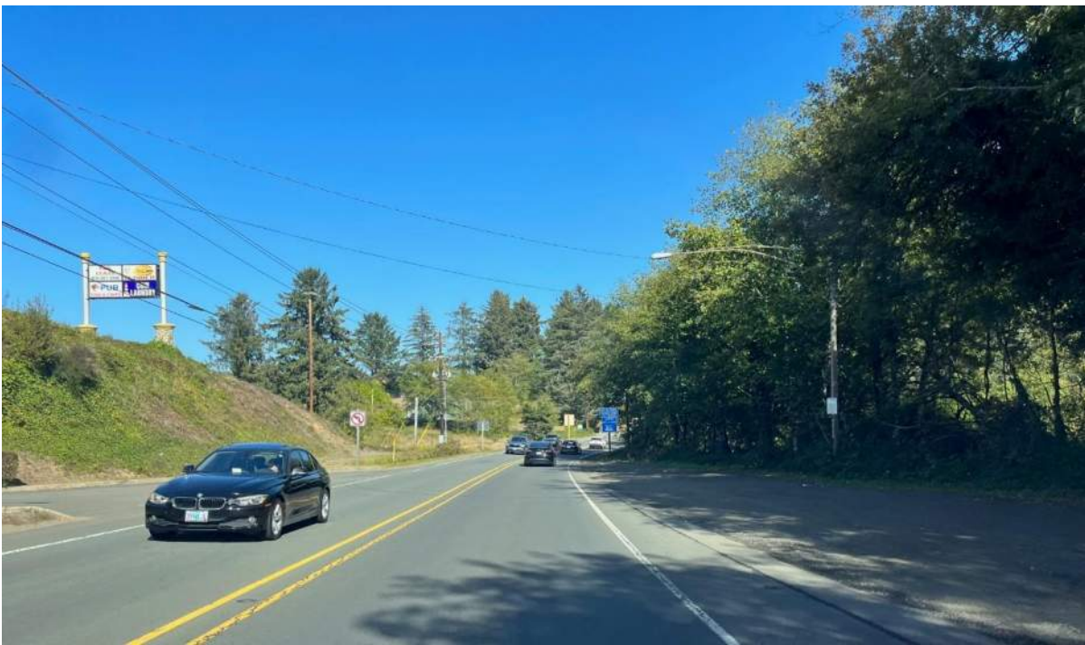
Figure 11. Stopping sight distance from 500’ south of the access. The access is visible, but partially blocked by the tourist information sign.
