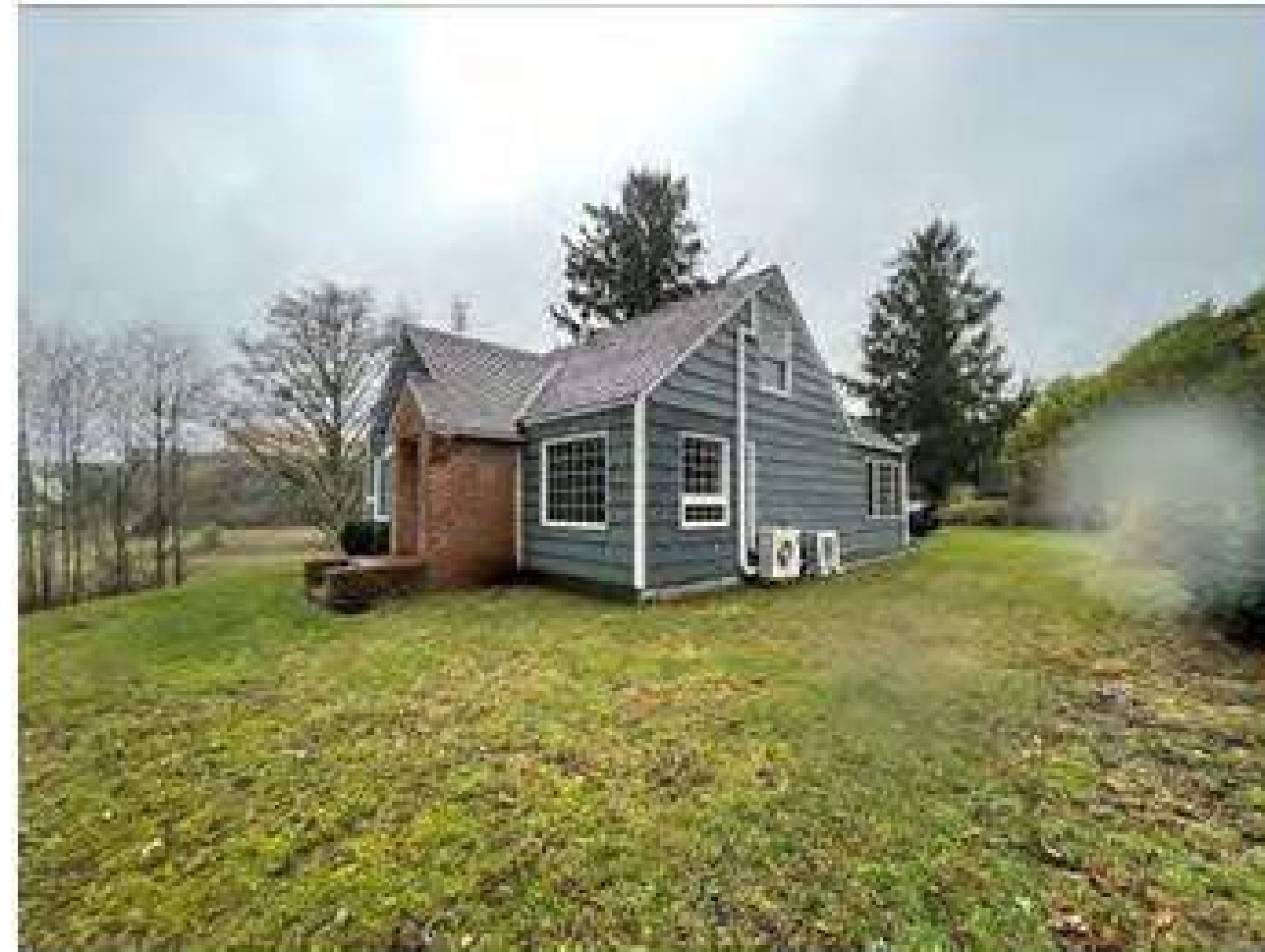
Existing Home SEC Facing NW
