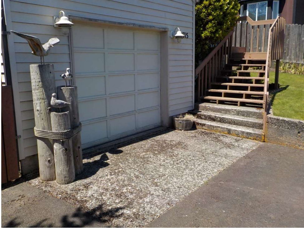
Photo 5 – View of the east side of the garage and driveway.
