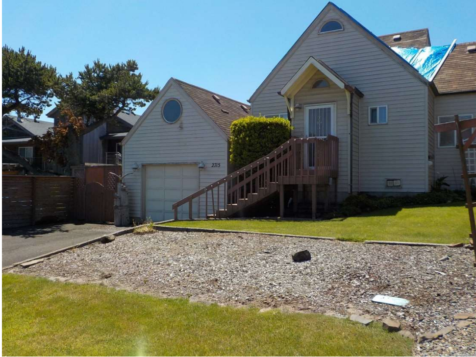
Photo 1 – Southwesterly view of 2715 NW Inlet Avenue from near Inlet Avenue.
