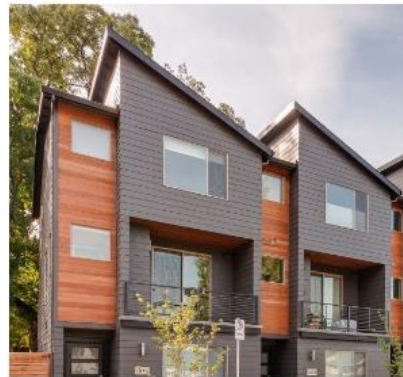
Roof line and building face offsets, and recessed balconies.
