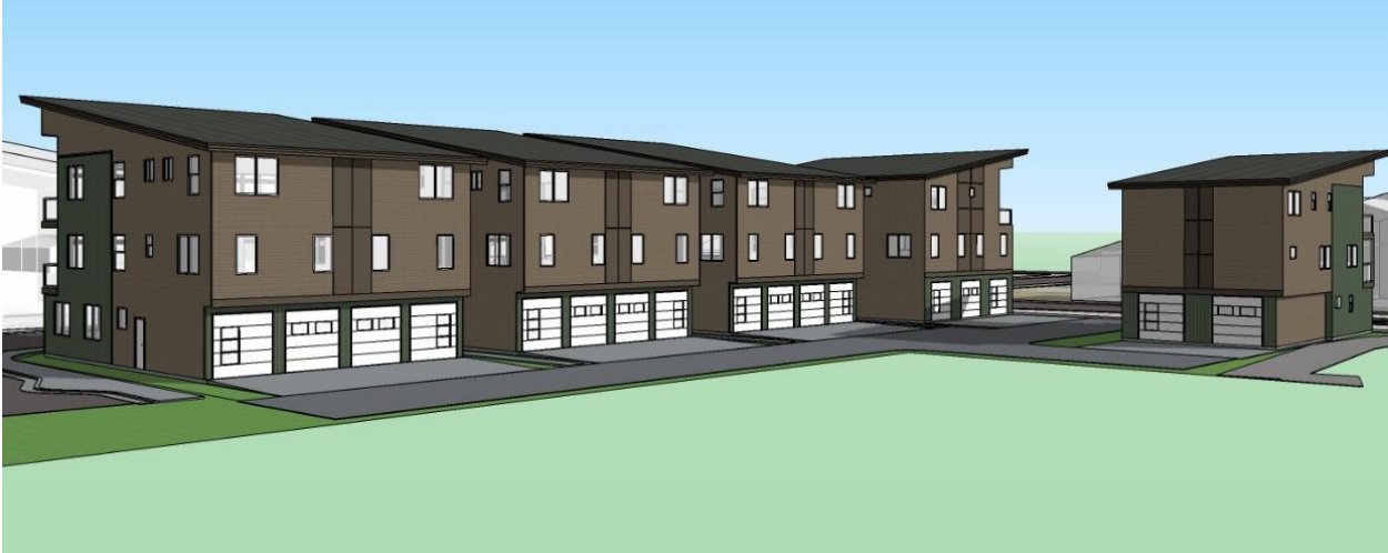
Looking southeast toward the interior of the development.
