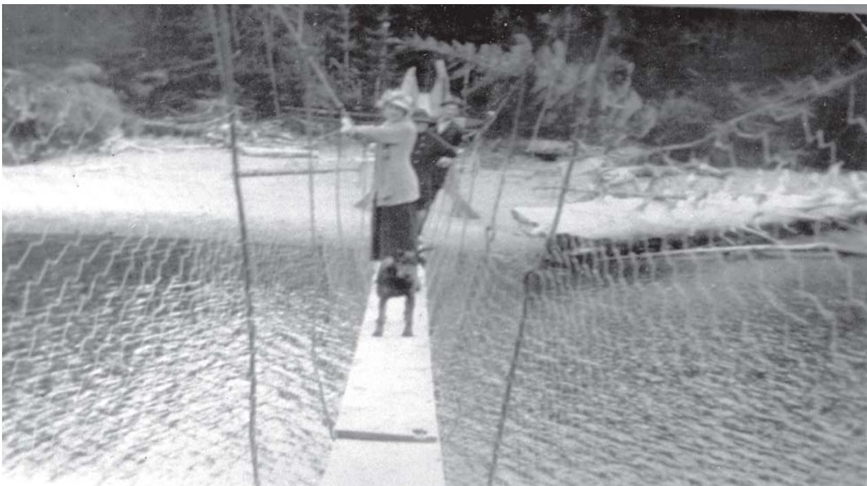
Bessie Knauf and Hazel King crossing Schooner Creek swinging bridge
